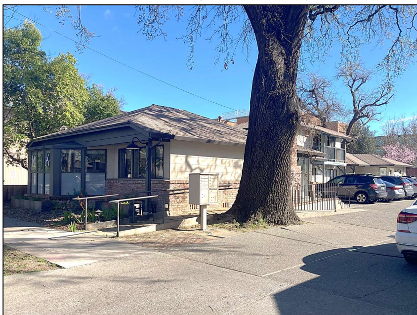
P5b. Description of Photo: Primary (west) and secondary (south) façades, view facing northeast. March 7, 2024.
