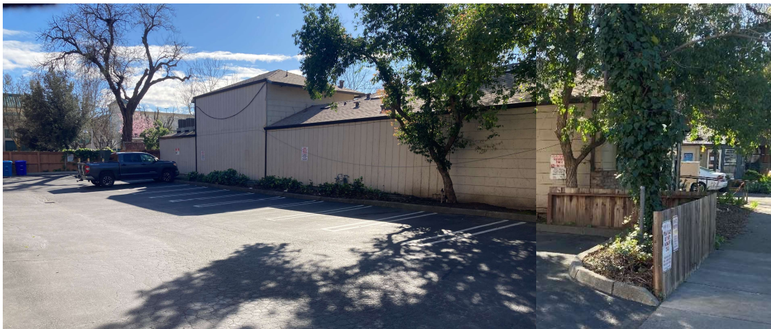
Rear (north) façade, composite view facing southeast. Source: ESA, 2024.
